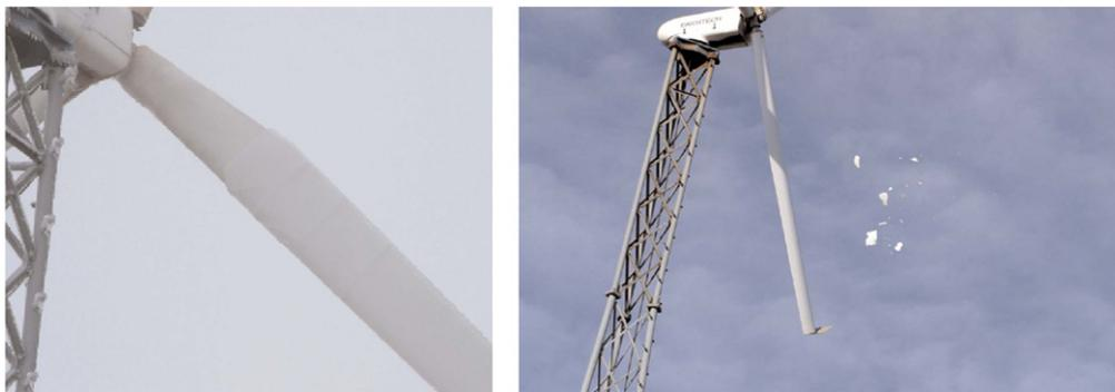
**Figure 6.** Ice accumulation and falling off on a wind turbine at Wachusett Wind Power (Windaction 2012).
